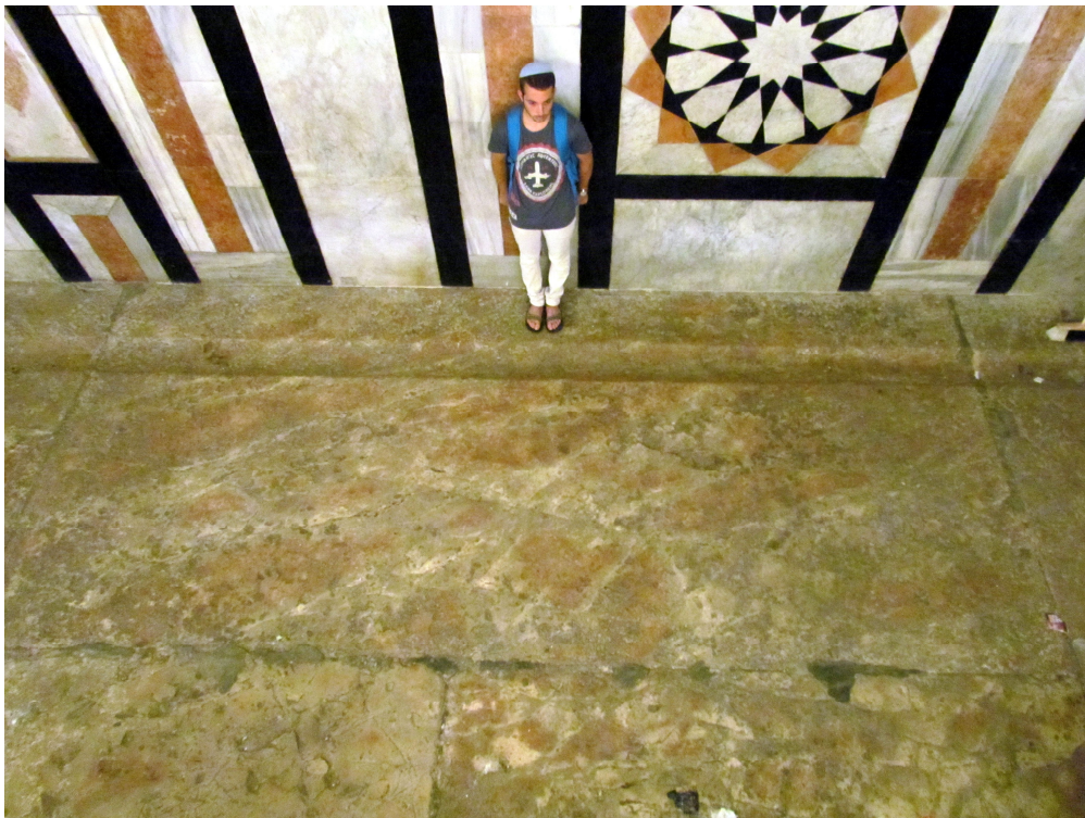
Fig. 3: The second largest paving stone: length 5.26 m., width 2.37 m. Note the gutter.
